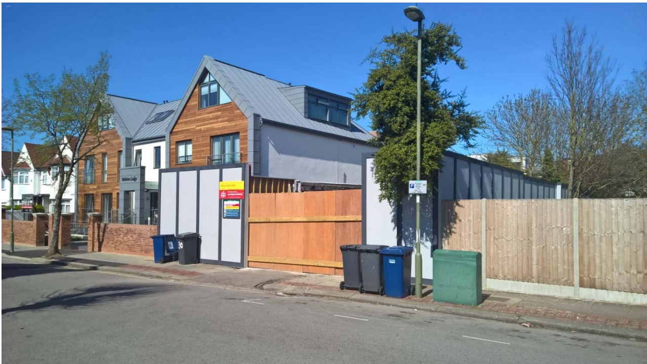
Figure 1 - Site access from The Grove
