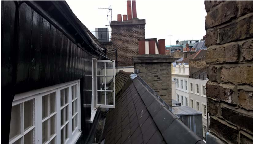
Roof scape – looking West to No43 and beyond
