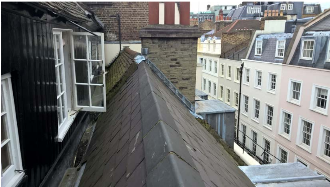
Roof scape – looking West to No43 and down
