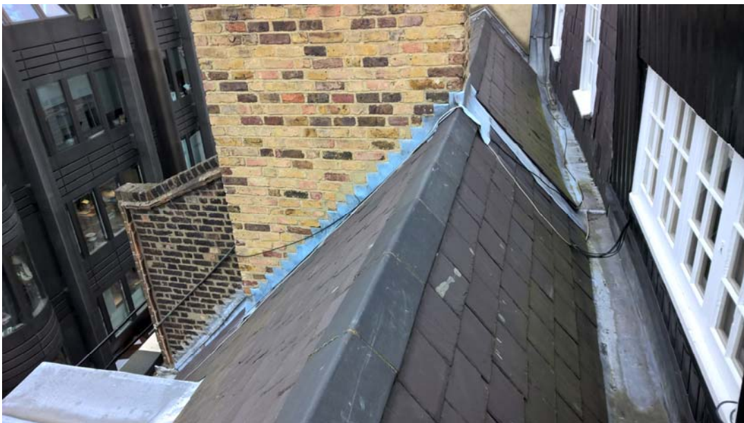
Roof scape – looking East to No45 and down
