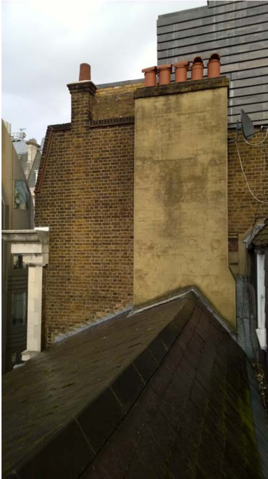
No45 – adjacent mansard conversion
