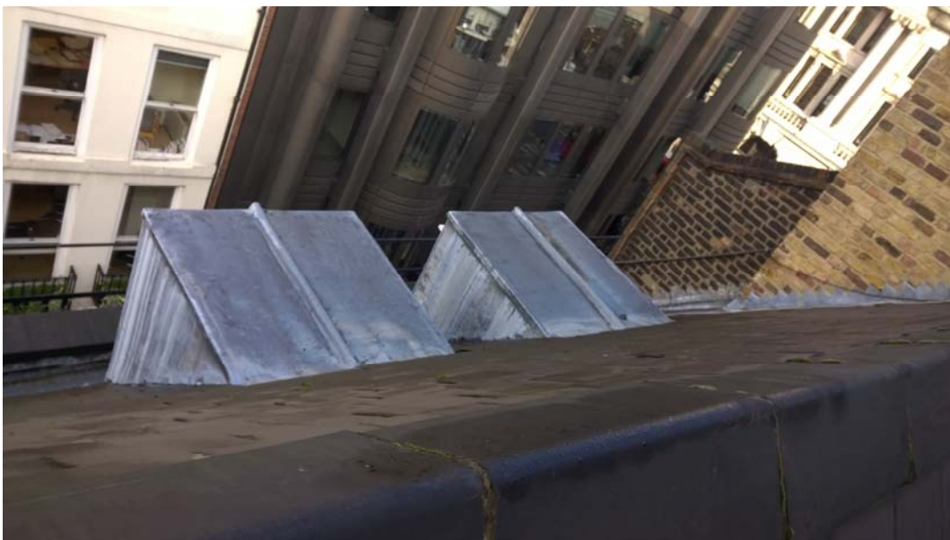
Existing roof with dormers and extended boundary wall No45
